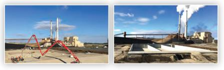
separated by internal 14-foot-tall walls, 24 inches thick as well. COP Construction placed more than 6,200 cy of concrete and the iron workers placed 2,000,000 pounds of rebars in a span of three months. A 780 cy mud slab was poured once subgrade was made to allow for a clean worksite during wet conditions. The concrete slab and wall pours had to be sequenced so that adjacent placements were not placed within seven days of each other.
