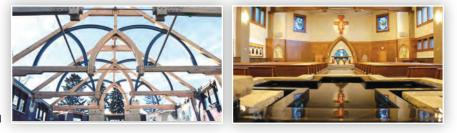
renovation/restoration. The project involved nearly three miles of wood base, casing and extension jamb molding, trusses that were a merger of steel and wood that span more than 68 feet, and much more. While portions of the building were demolished, various face stones were salvaged and incorporated into the new walls. Crews worked in close coordination to manage limited available space on the site and equipment size restrictions.
