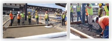
project was the incorporation of a pervious concrete parking lot rather than utilizing asphalt in areas where no large equipment will be driven. To date, this is the largest pervious placement in Montana, consisting of 655 cubic yards. White Resources LLC placed the pervious concrete in four rather than the anticipated five days, with the technical assistance of David Mitchell – Bunyan Industries.
